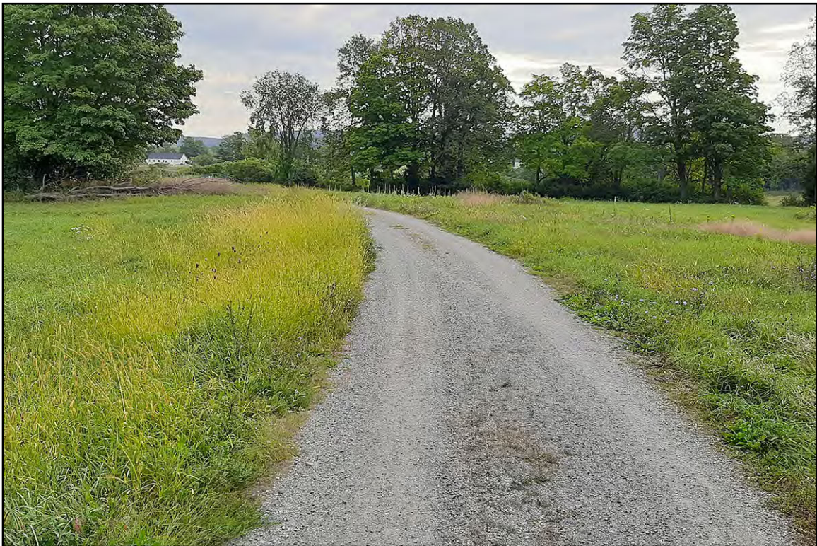
PLATE 89: Access Road Between Structure 306 and Brigham Road
