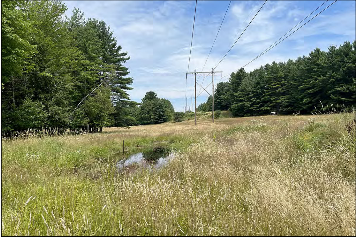
PLATE 27: Structure 396 and Wetlands, View North
