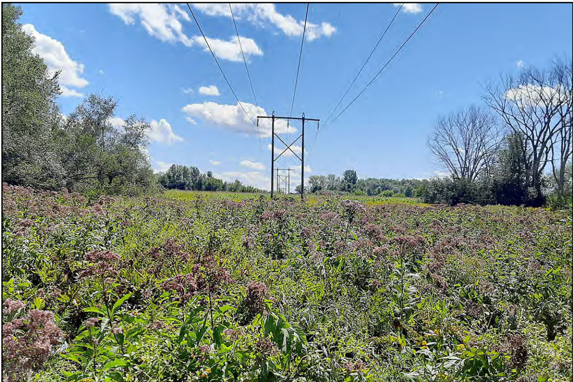
PLATE 121: Structure 248, View Southwest
