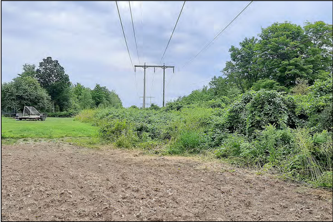
PLATE 96: Structure 291 with Surrounding Vine and Bramble Covered Bedrock, View West
