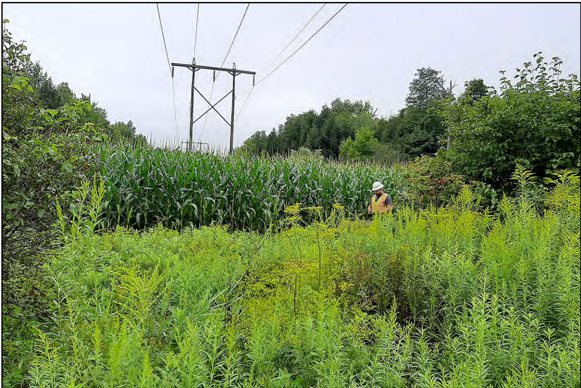
PLATE 138: Structure 232, View South
