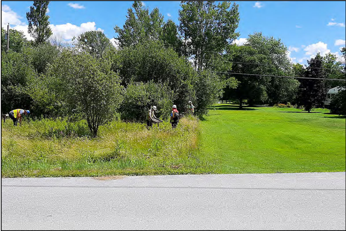
PLATE 54: Excavations South of Structure 357, Standing Water in Lawn, View East
