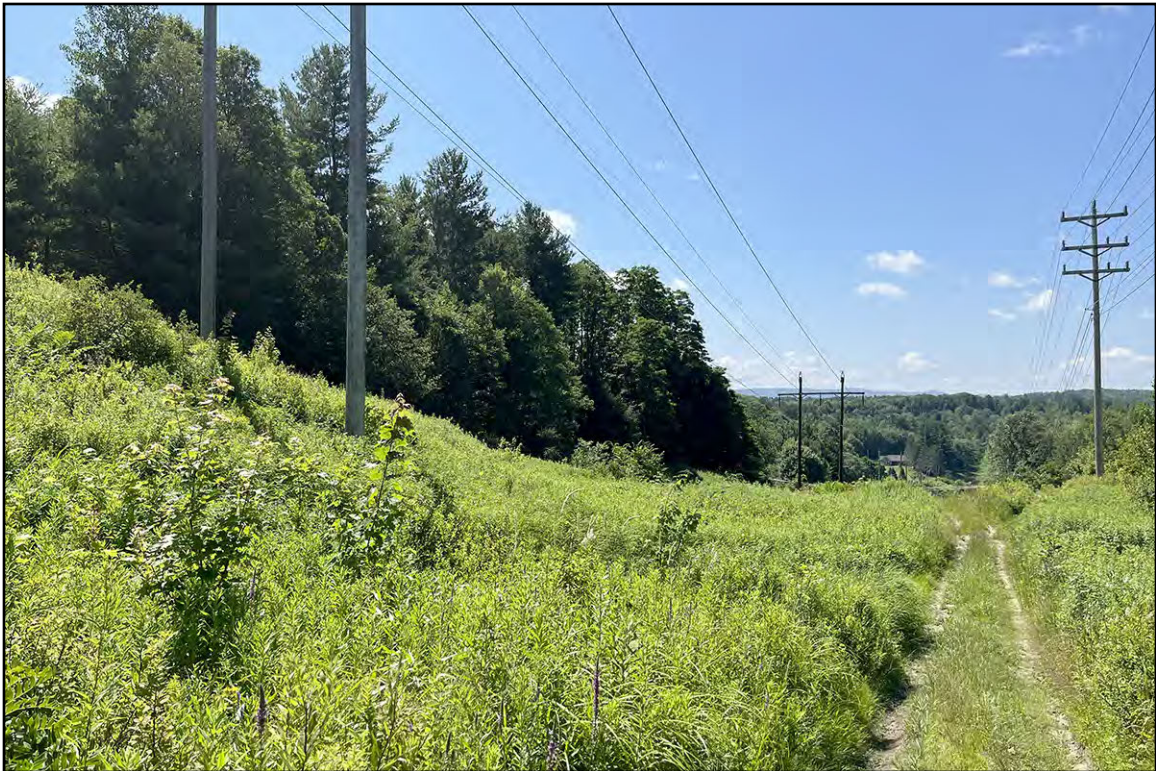
PLATE 6: Slope, Artificial Bench and Road at Structure 418, View South
