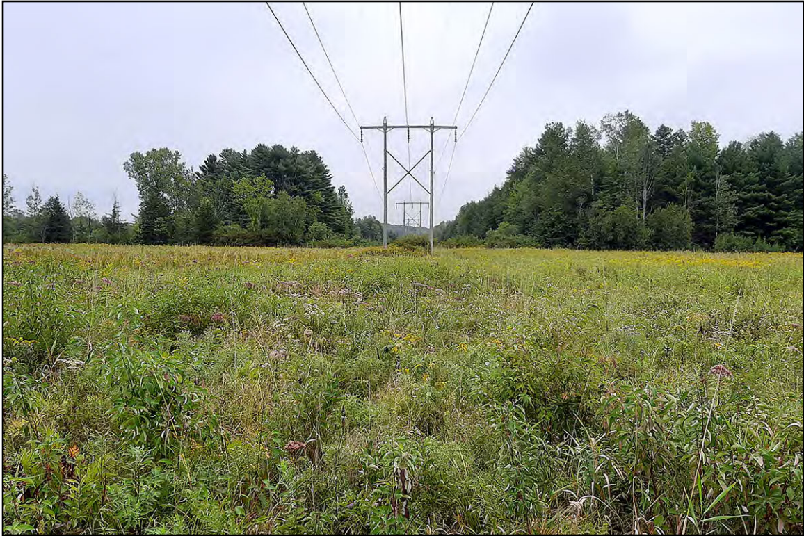
PLATE 112: Structure 257, View Northeast
