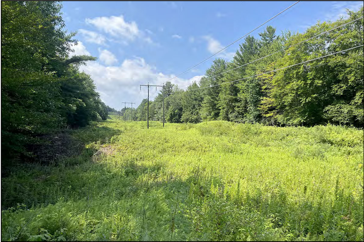
PLATE 25: Structure 405, View Southwest
