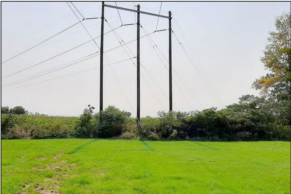
PLATE 75: Structure 329, View Southwest
