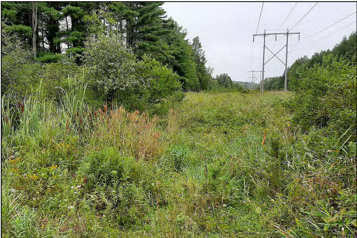
PLATE 111: Structure 258 and Area with Standing Water, View North
