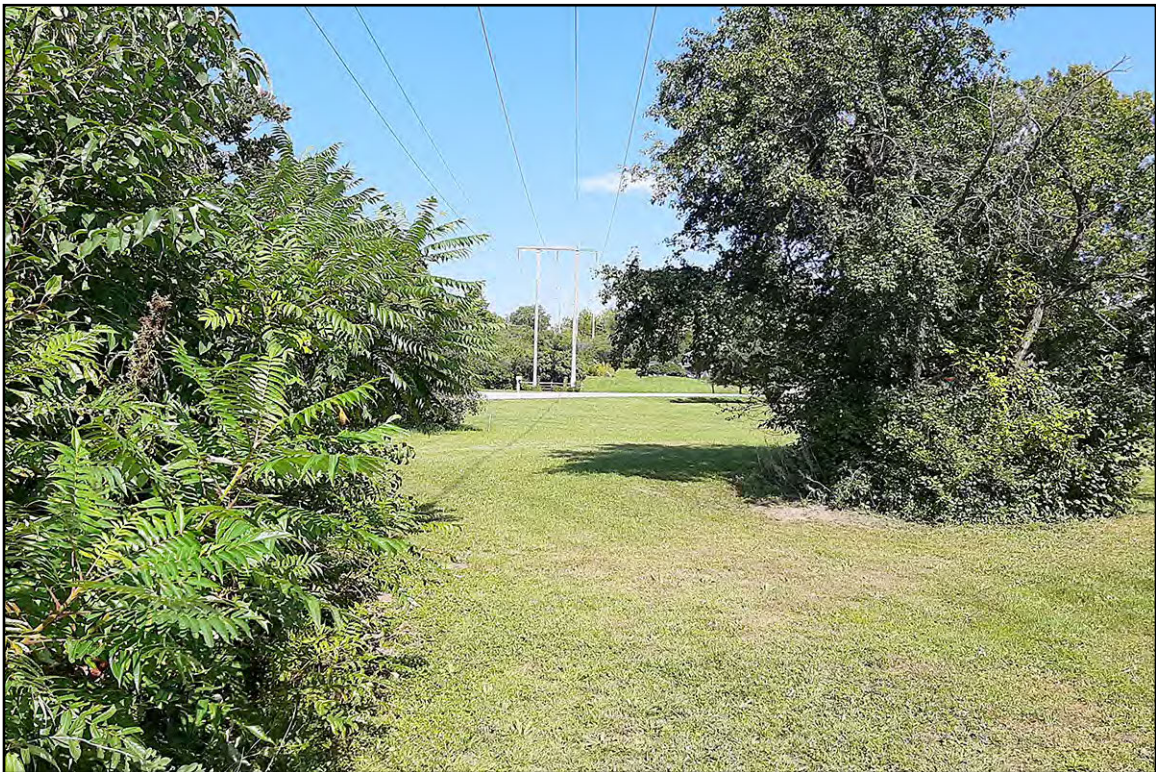
PLATE 62: Overview of Structure 350, View Northeast
