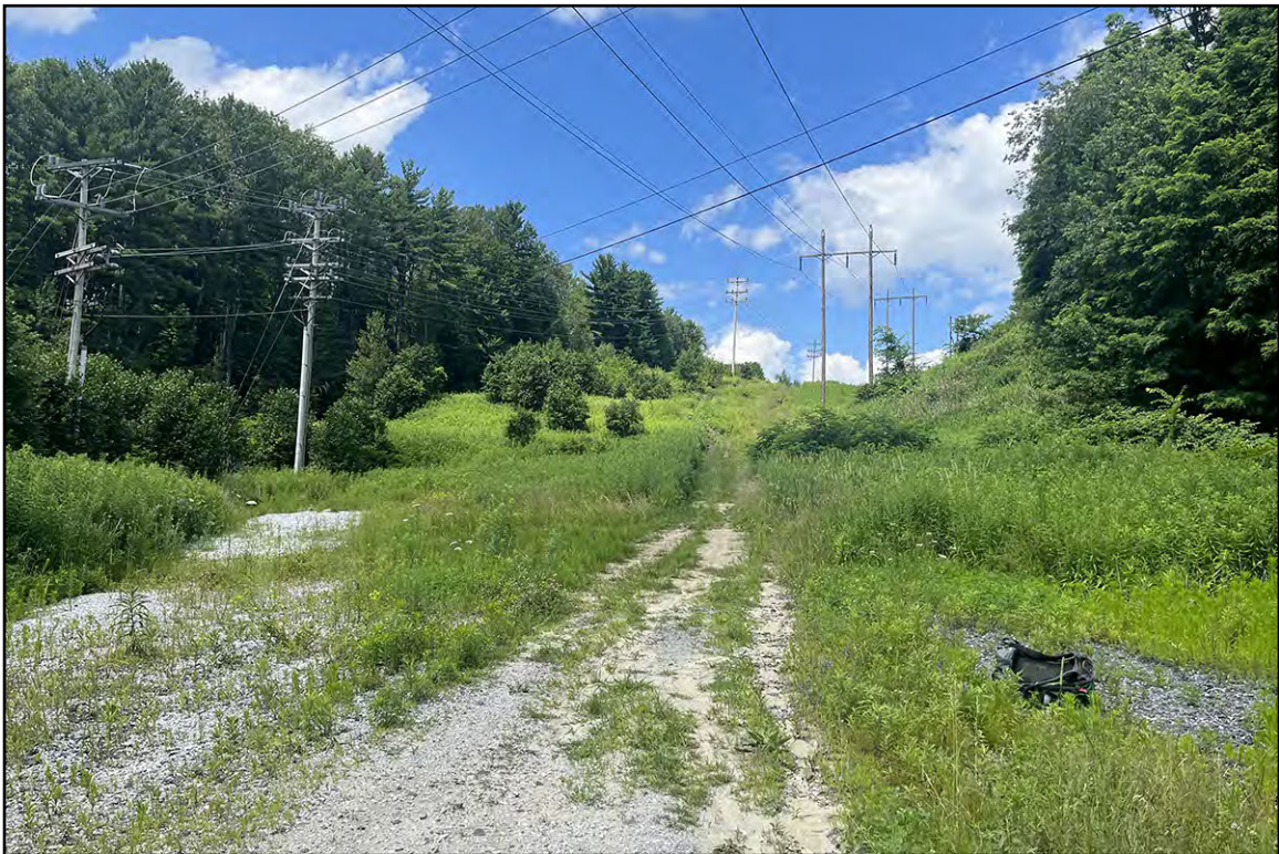
PLATE 12: Gravel Road East of Structure 416 to Structure 417, View North
