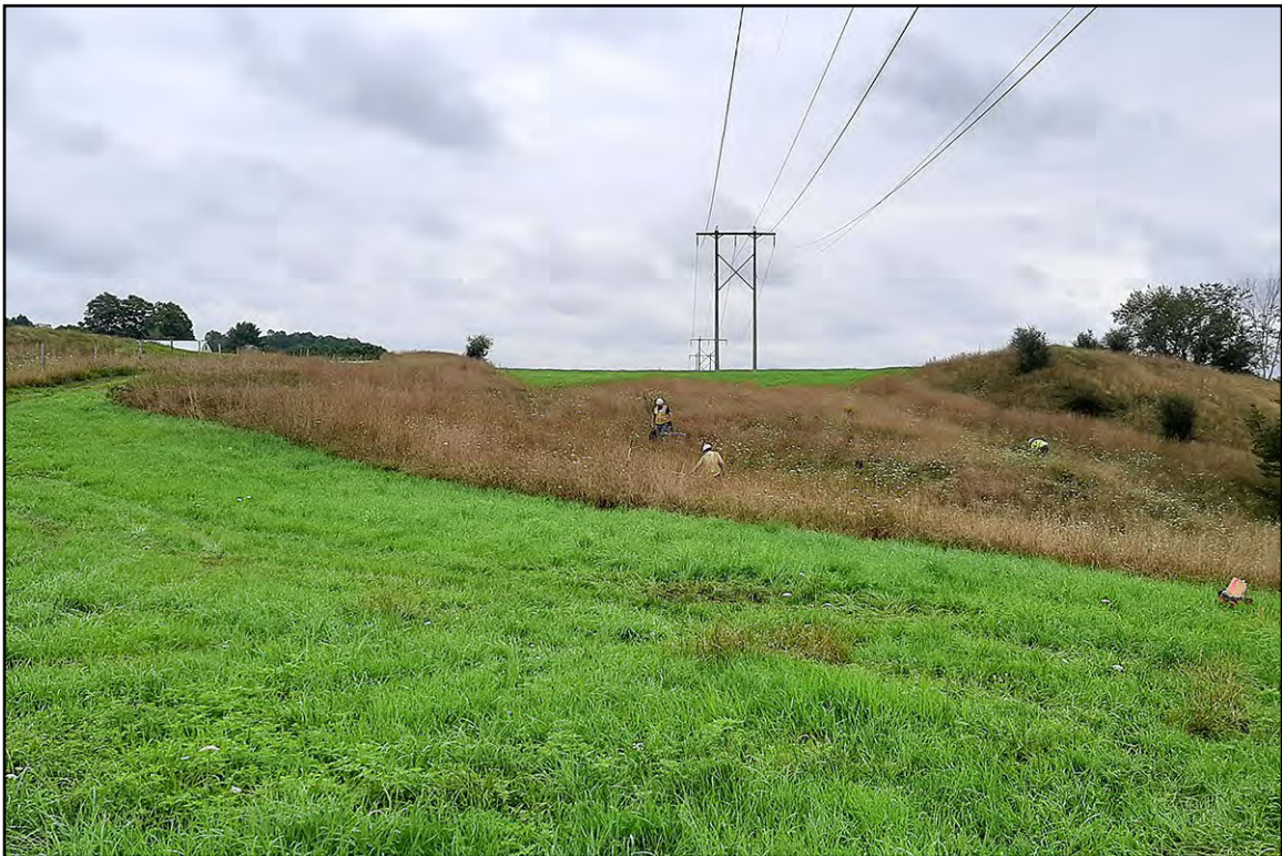
PLATE 144: Access Road South of Structure 226, View South
