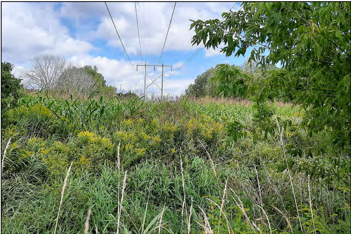
PLATE 119: Structure 250, View Northeast
