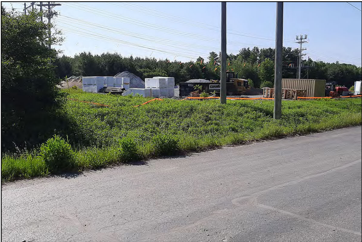
PLATE 5: Overview of Storage Area Between Structures 421 and 420, View Southeast
