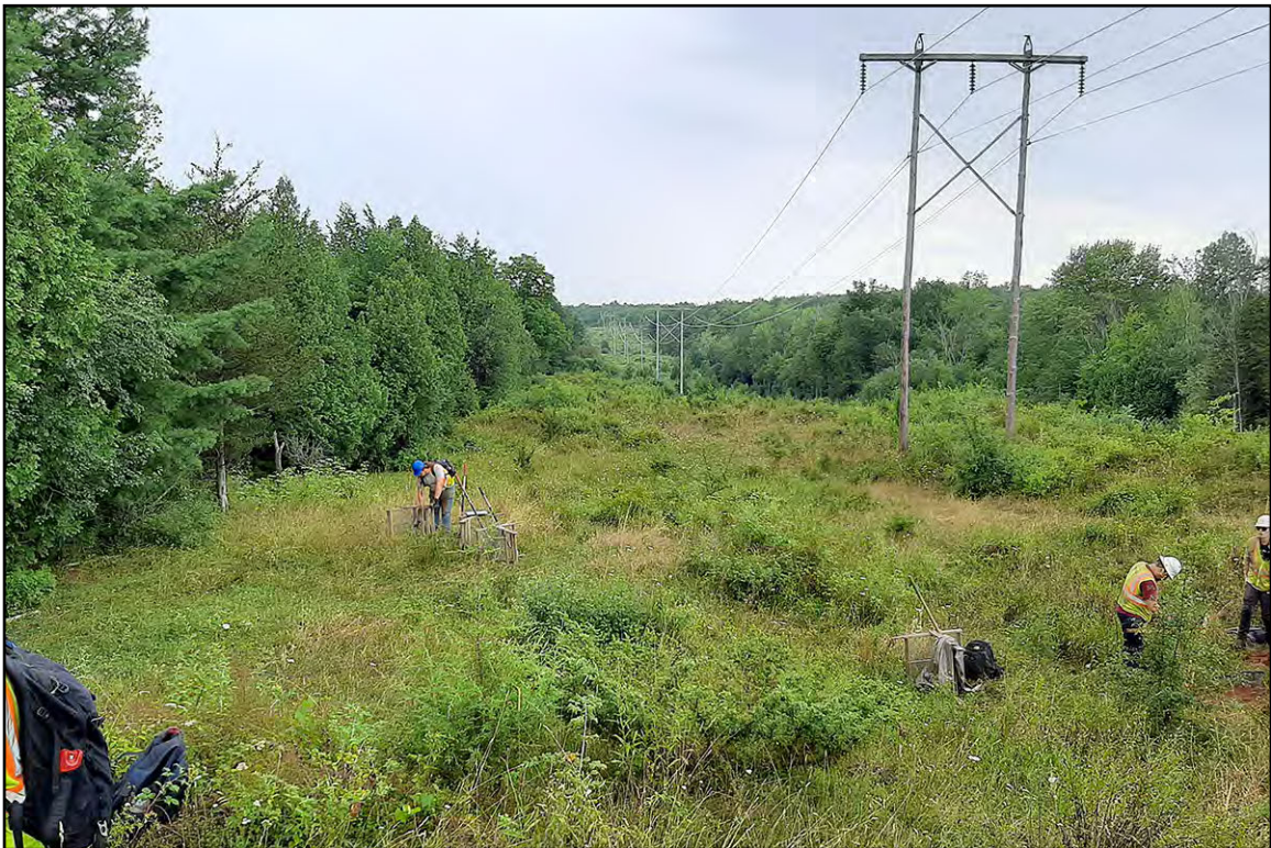
PLATE 99: Excavations at Structure 281, View South
