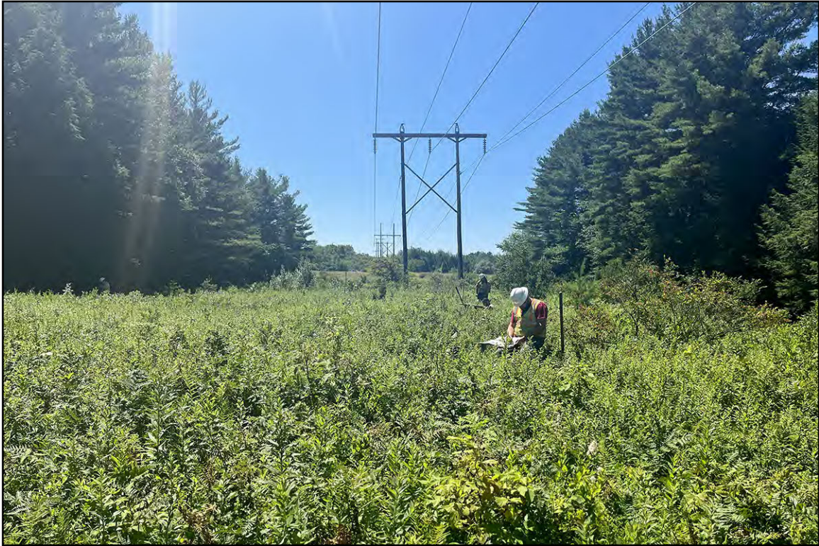
PLATE 31: Excavations at Structure 394, View North
