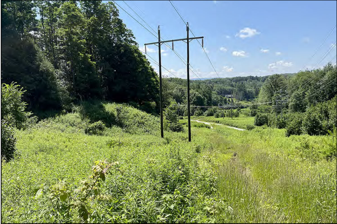
PLATE 7: Structure 417, View Southeast
