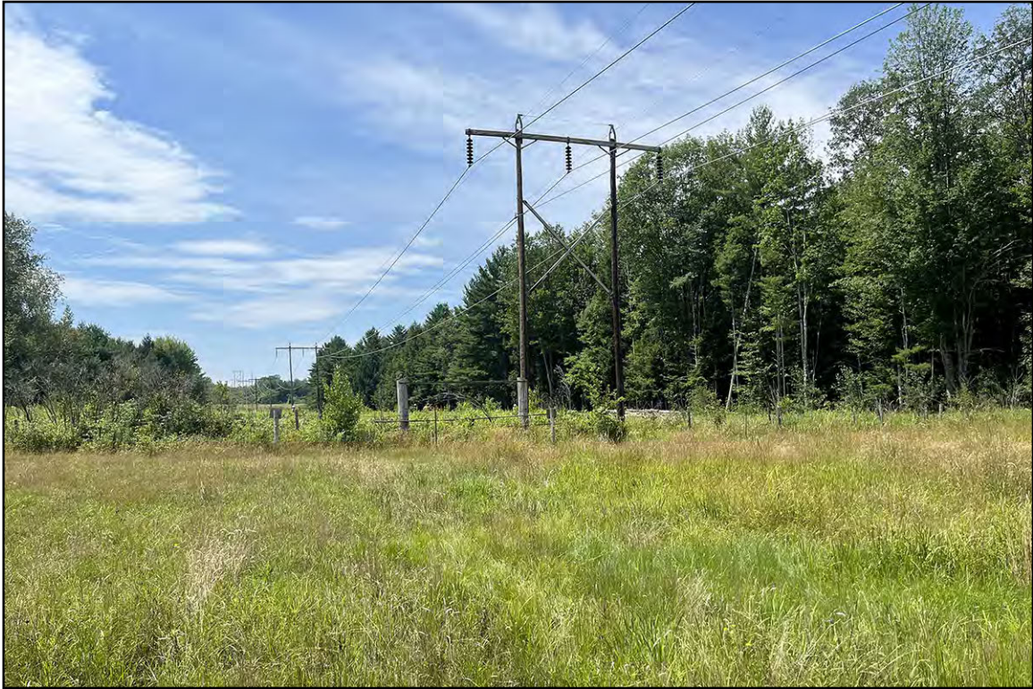
PLATE 29: Structure 395, View South
