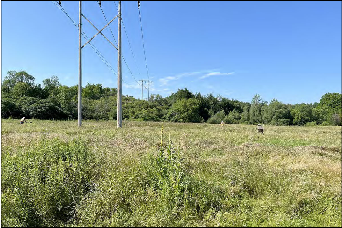
PLATE 33: Excavations at Structure 391, View South
