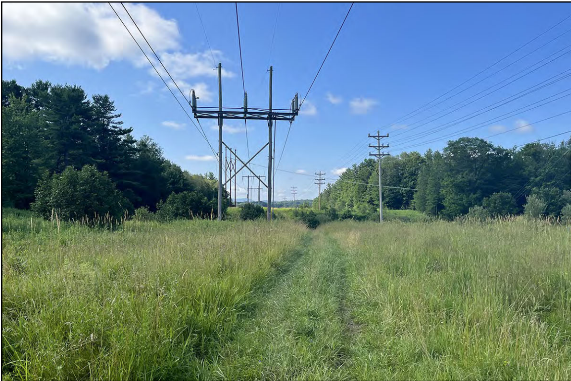
PLATE 3: Access Road Disturbance and Structure 420, View South
