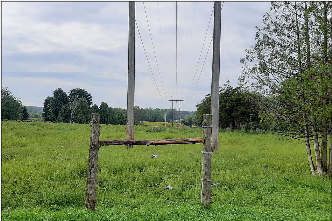
PLATE 106: Structure 268 in Fenced Pasture, View South
