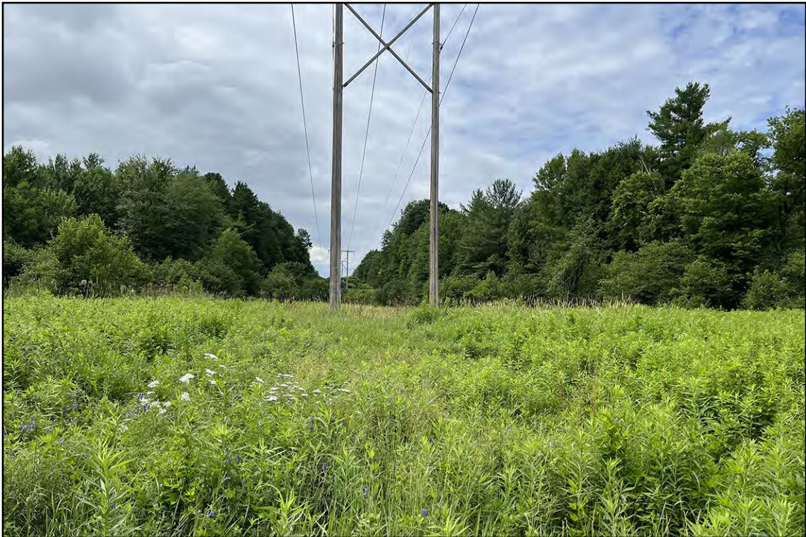
PLATE 20: Structure 412, View South
