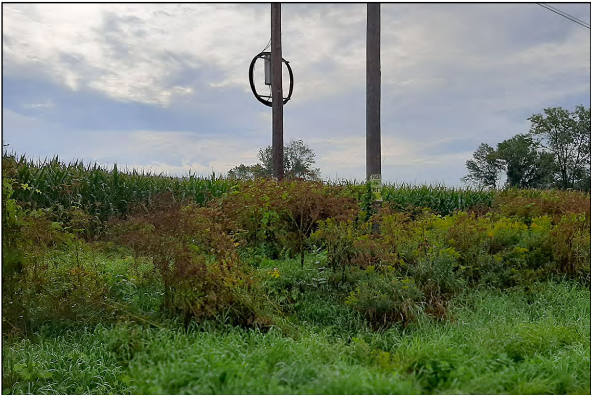
PLATE 108: Structure 266 with Ditch, Wild Parsnip, View East
