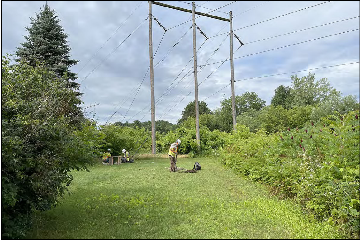
PLATE 14: Excavations at Structure 414, View Southwest
