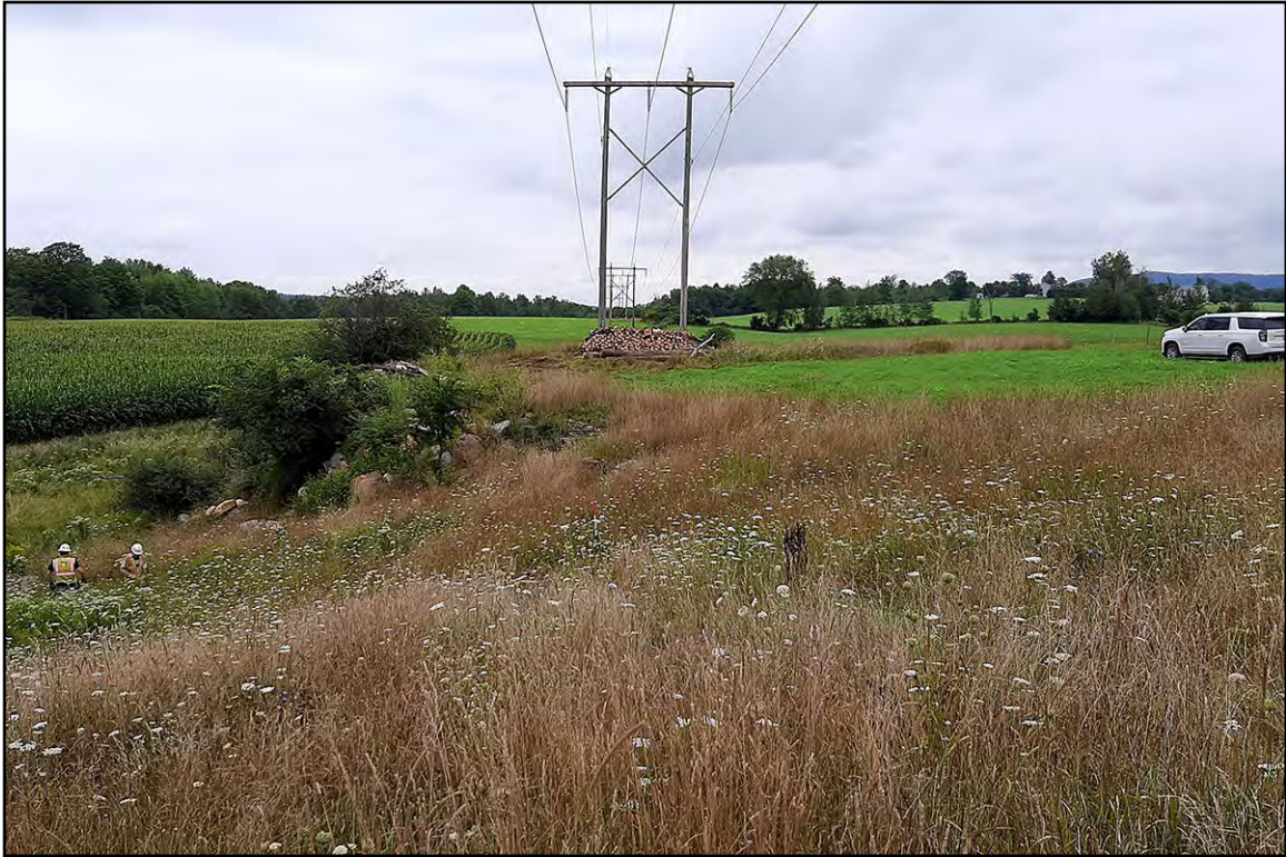
PLATE 143: Structure 226, Landowner Refuse Dump and Firewood, View North
