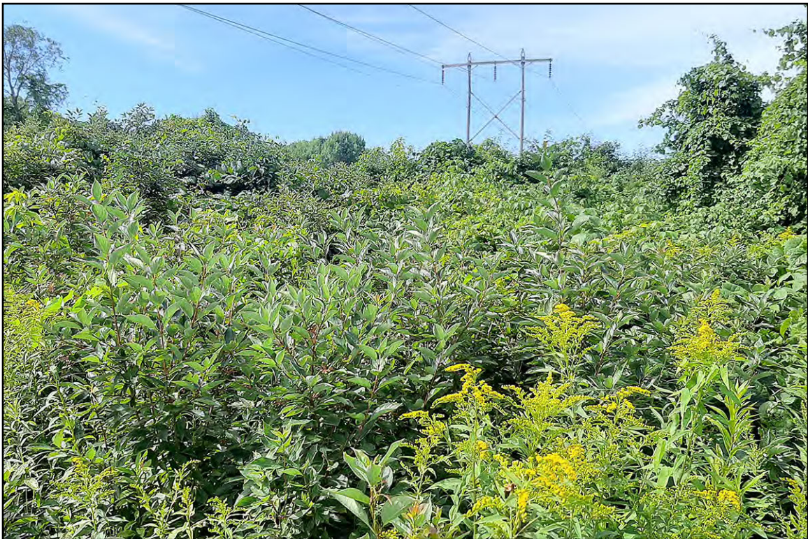
PLATE 69: Area North of Structure 337 Blocked by Shrubs, Vines, and Brambles, View Southwest
