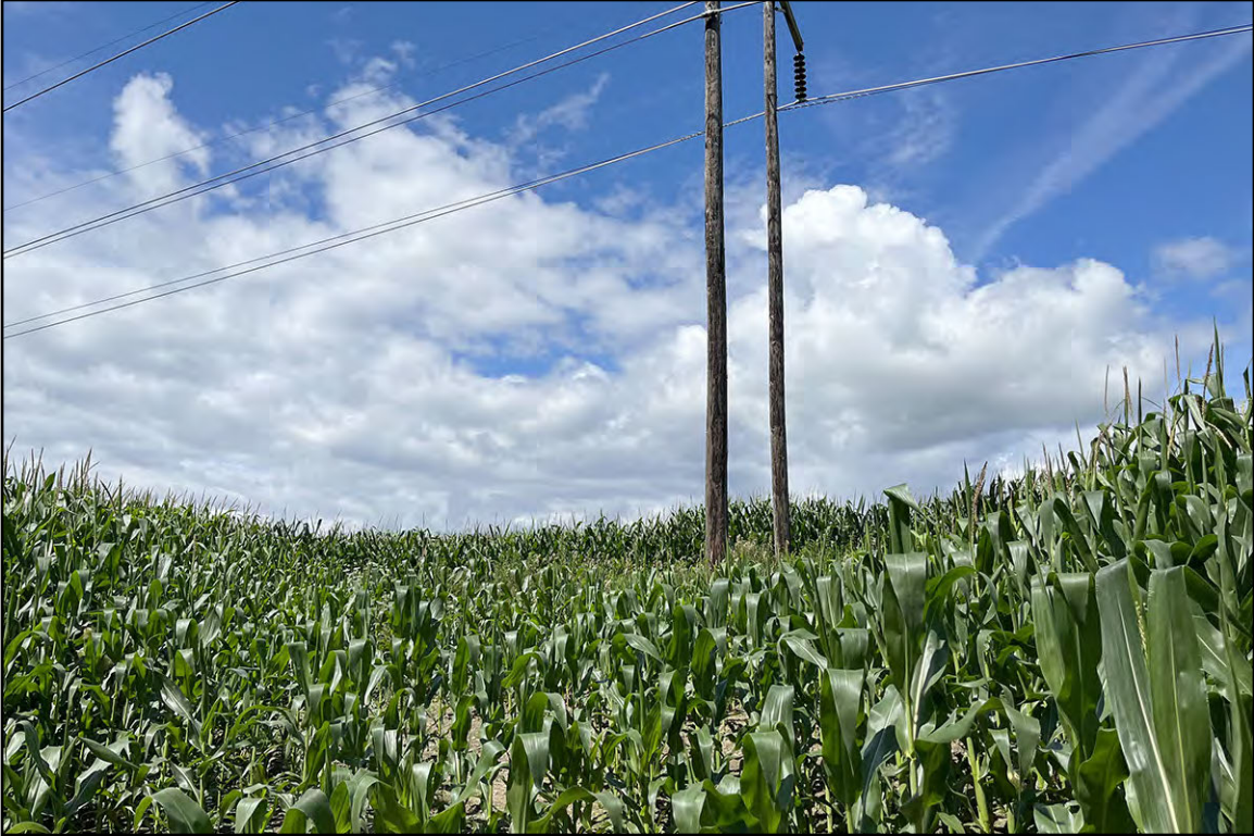
PLATE 42: Structure 380, View West
