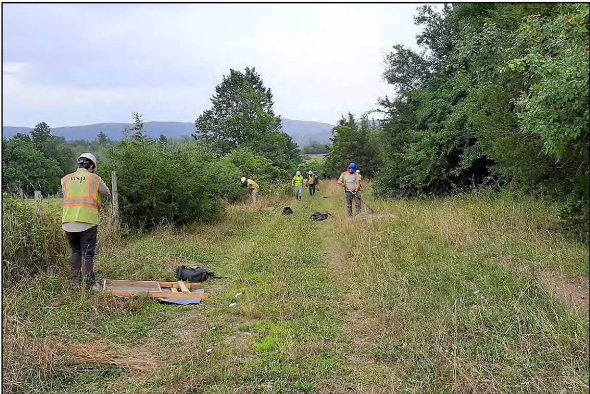
PLATE 97: Excavations Along Access Road from ROW near Structure 284 to Bronson Road, View South
