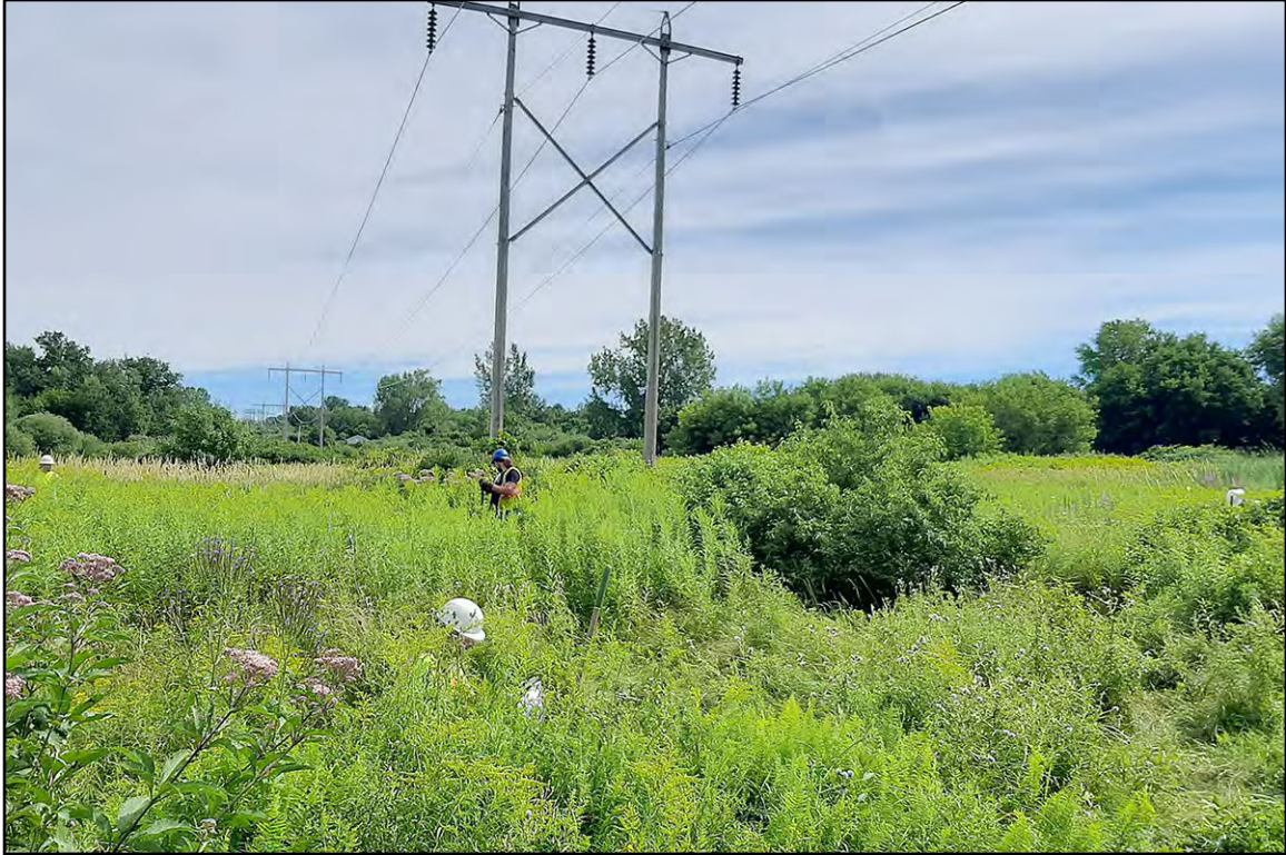
PLATE 68: Excavations North of Structure 338, View East
