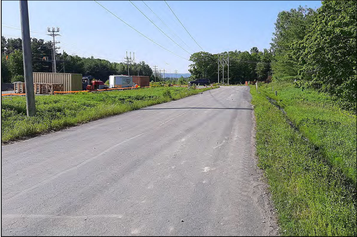
PLATE 4: Overview of Storage Area Between Structures 421 and 420, View South
