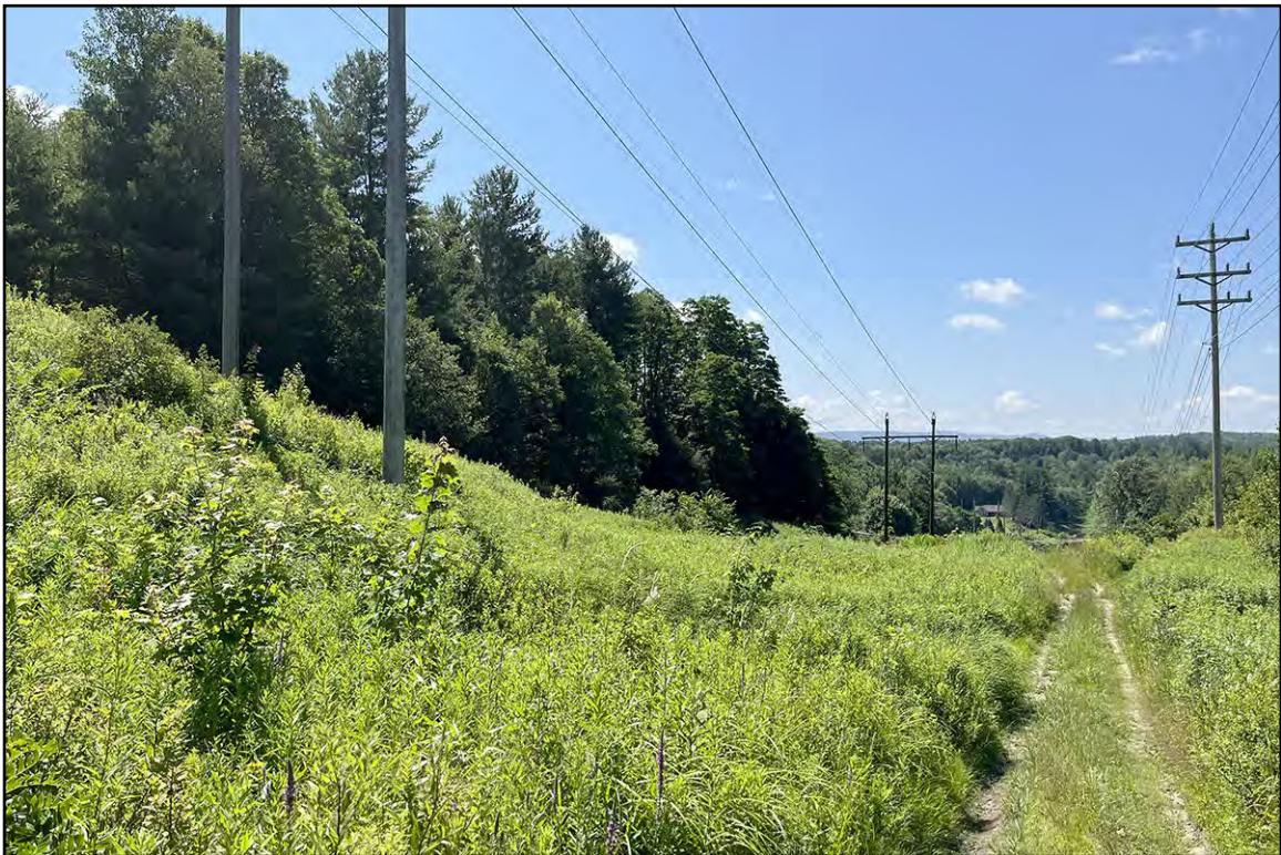
PLATE 8: Slope and Erosion near Structure 417, View North
