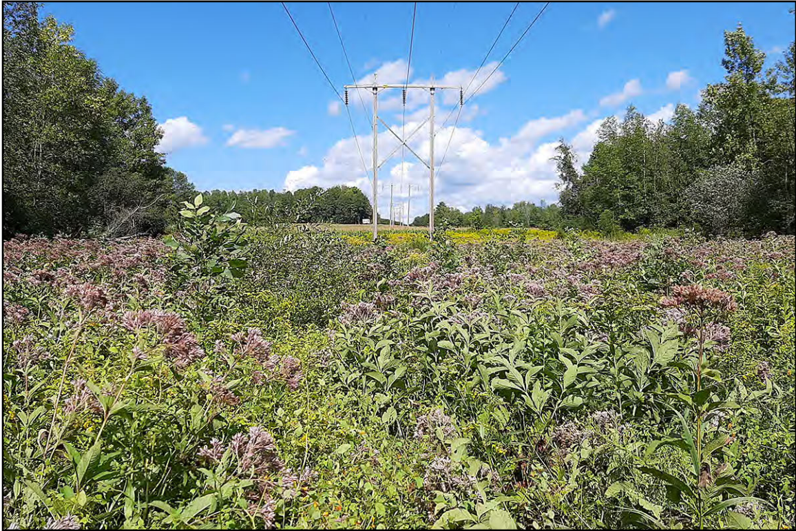
PLATE 120: Structure 249, View Southwest
