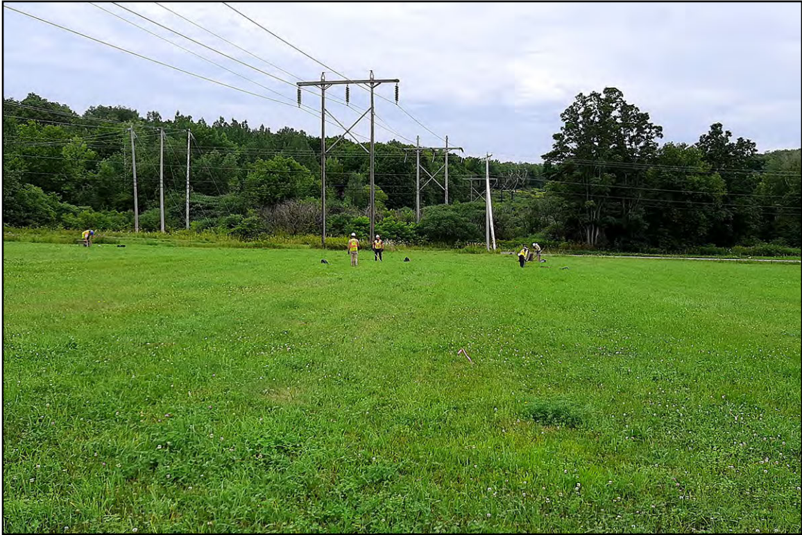
PLATE 92: Excavations at Structure 297, View South
