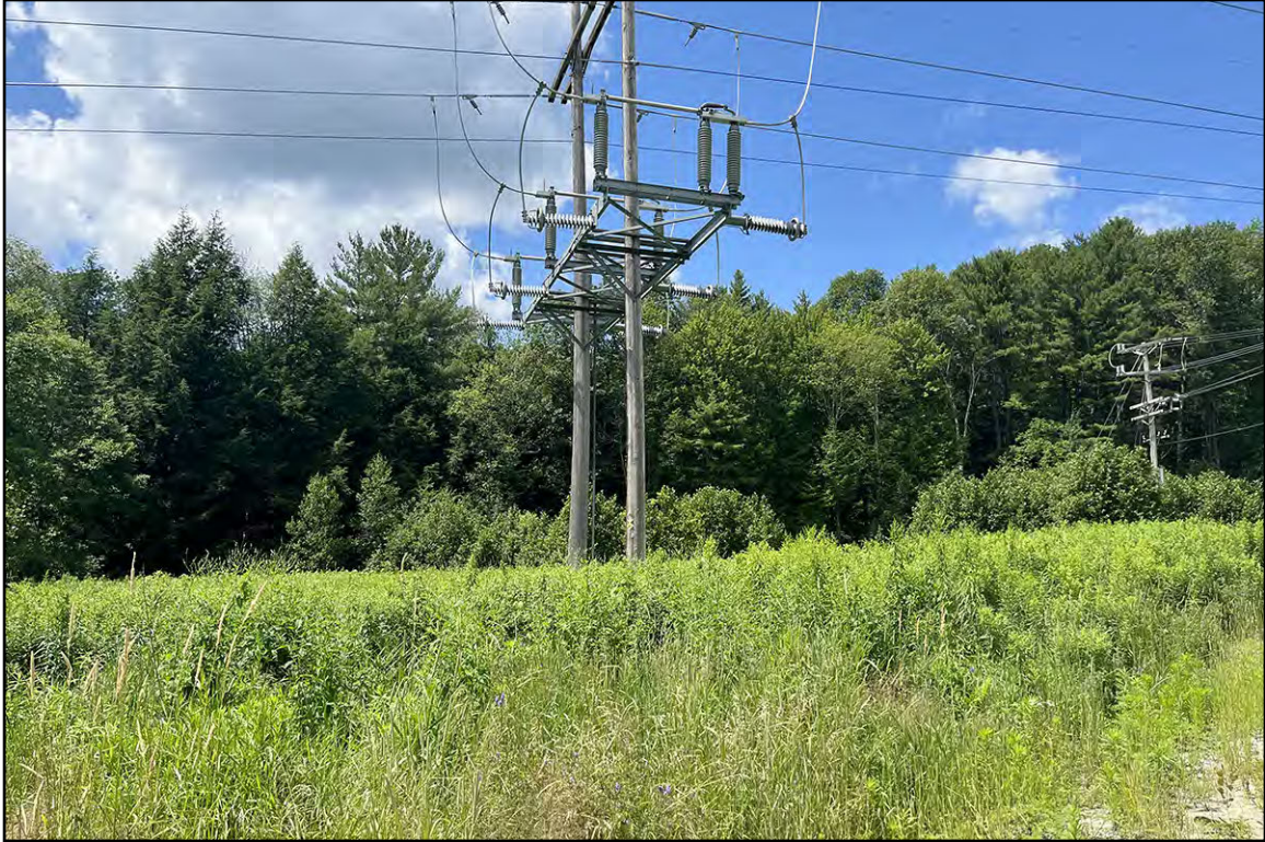
PLATE 9: Structure 416, View West
