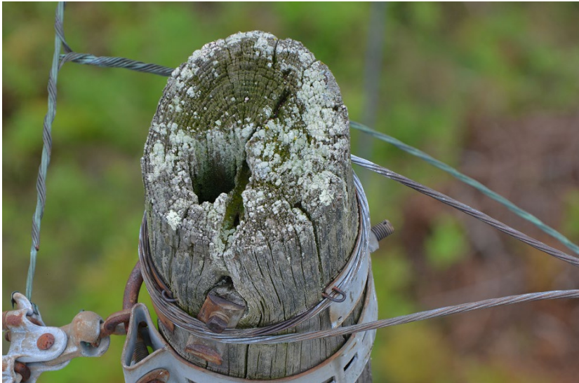
Examples of rotted pole tops
