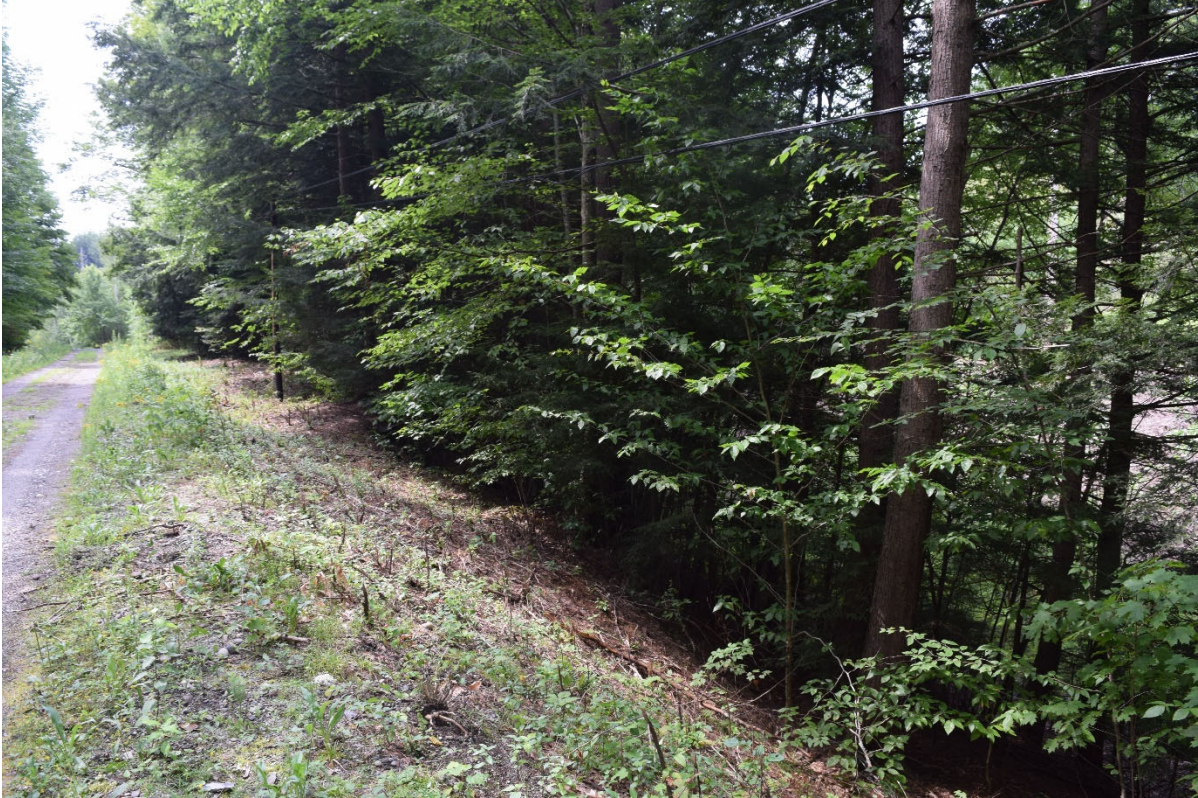
Photo 7. Steep embankment on west side of access road, view southwest.
