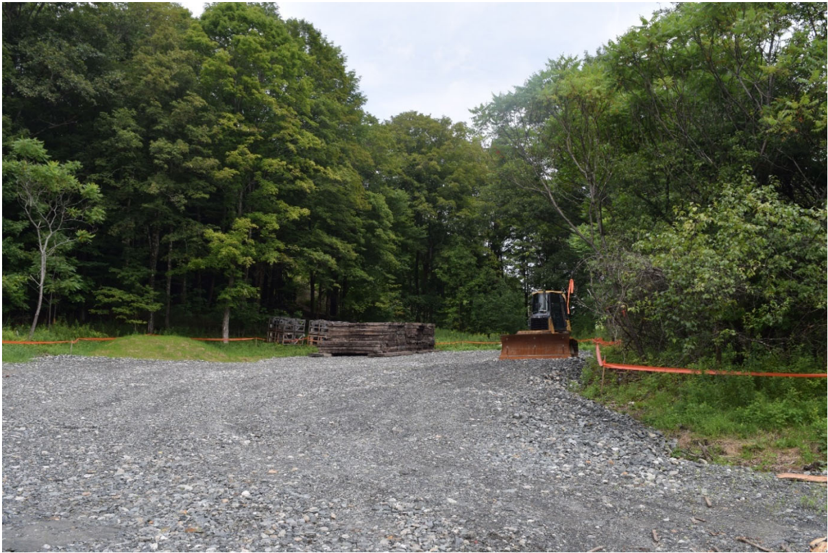
Photo 4. Laydown area, view southeast.
