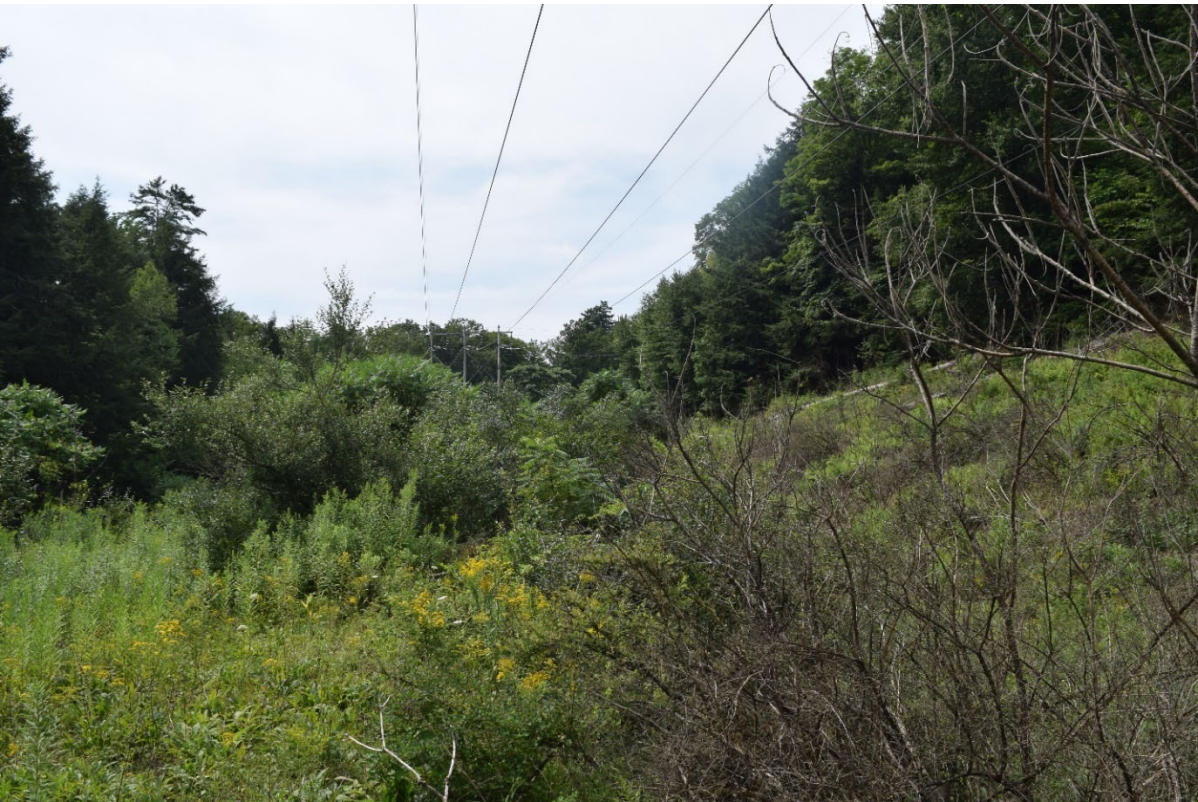
Photo 8. Transmission line right-of-way from substation, view southwest.
