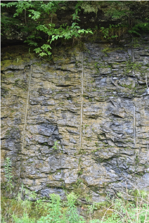
Photo 10. Quarry blast holes along the east-facing bedrock ledge face, view west.
