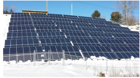
Figure 23: This is a photo of the Town-owned 150 kW solar project in Cavendish as described on page __. This is an example of a perfectly sited project. Because it is not visible from any major public roads and has no neighbors, no landscaping is warranted. (Credit: Peter LaBelle)
