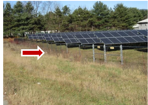
Figure 24: This project is an example of inadequate landscaping/screening. Note deciduous shrubs do not provide year-round screening, small plants will take many years to grow up to provide effective screening, and a lack of mowing the grass between the landscaping and roadway, which is to the left of the photo.
